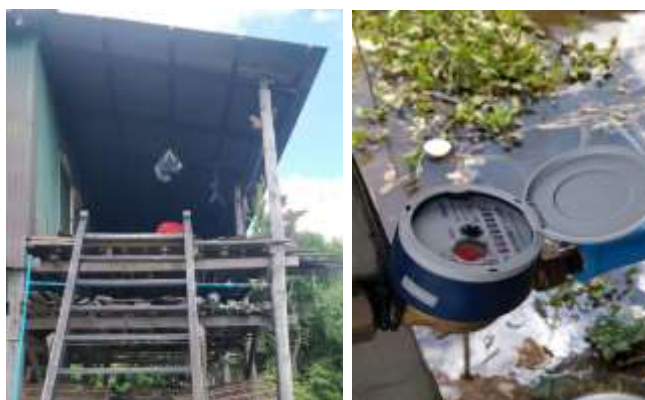
Photo 57: Piped water connection for poor households in S'ang district
