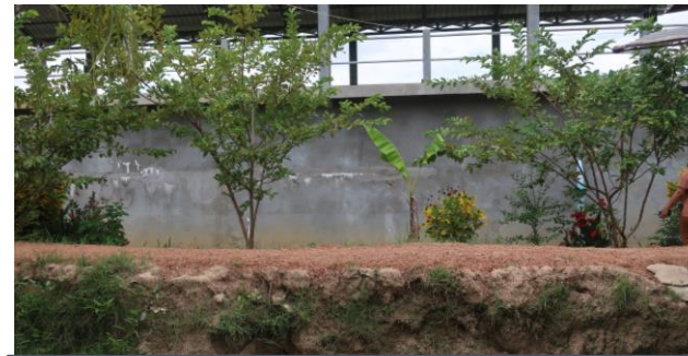
Flood protection for pipe water treatment plant
