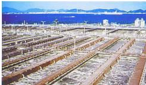
Development of sewerage
